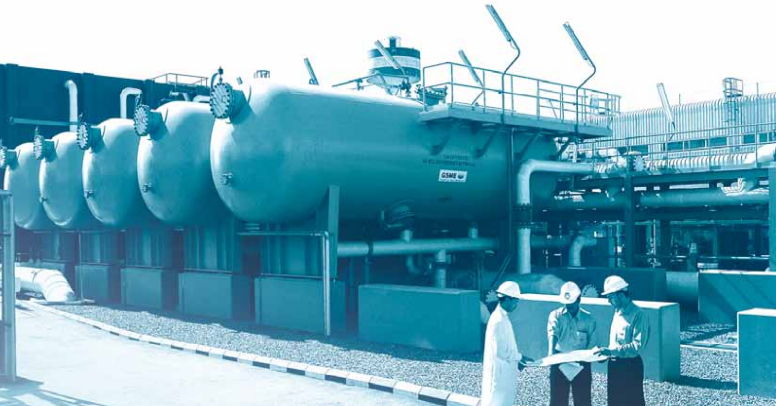
50,000 m 3 /day seawater membrane filtration system
